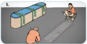
Apply the adhesive evenly on the installation place (SBR, concrete or tarmac).
